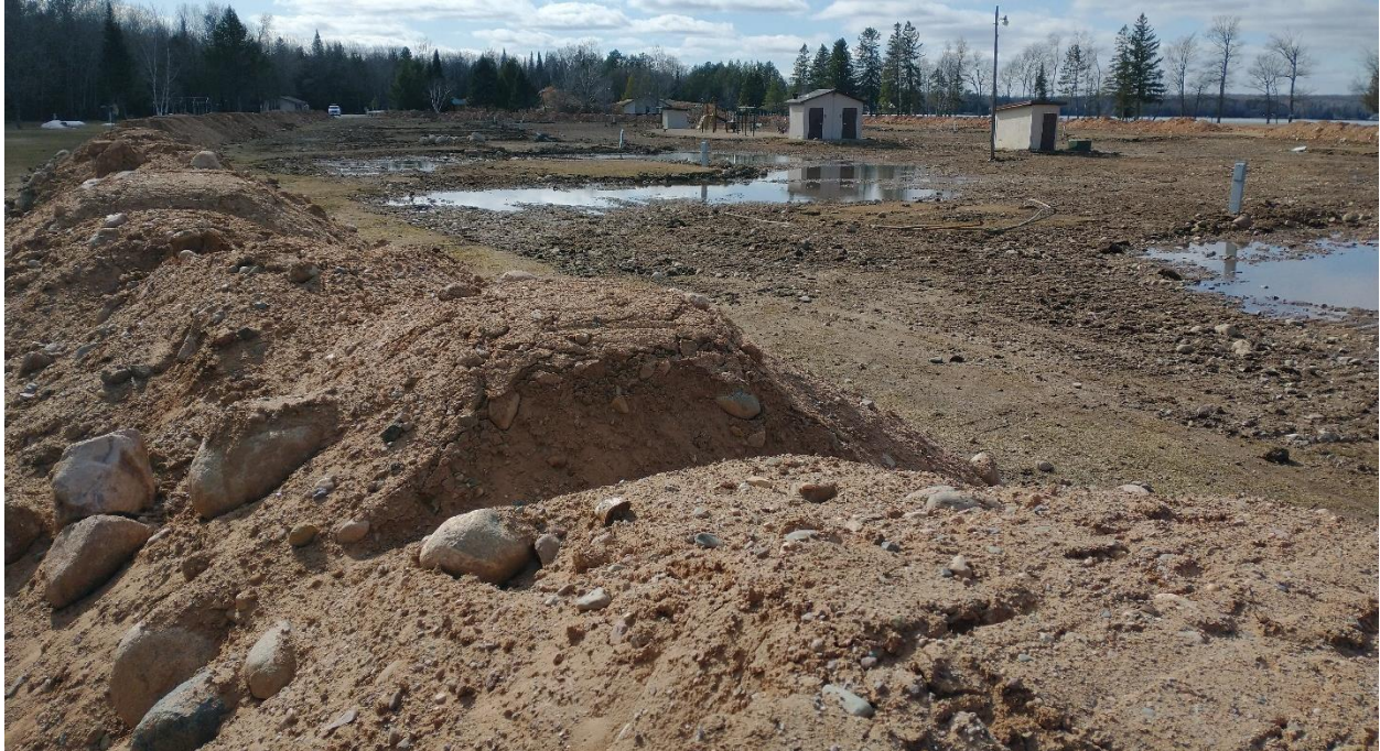
Photo 5 – Topsoil scraped central campsites and road (under fill material) from southeast of Project Area facing northwest
