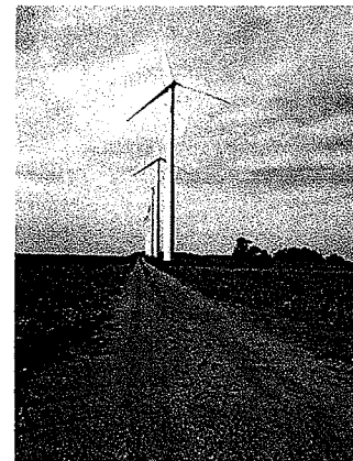
An access road leads to turbines in the WPS wind farm off of Pheasant Road at the Town of Lincoln in Kewaunee County, Wis. The turbine roads double as field access for farm equipment.
