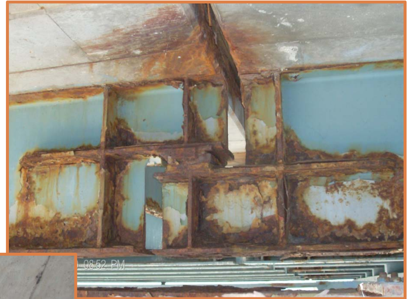
Corroded ship laps
