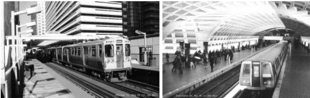
Heavy rail rapid transit trains can serve either elevated stations or underground subways within densely populated central cities, as illustrated by the Chicago Transit Authority “El” train (left) and Washington, D.C. Metro subway station (right). Service outside the central city is often above ground in freeway medians or other fully grade-separated rights-of-way.
