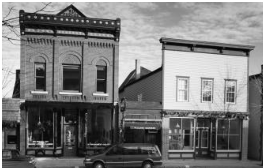
The Wisconsin Department of Commerce administers the Wisconsin Main Street Program in which the state provides assistance to local communities to revitalize their historic downtown business districts. These two stores in Dodgeville benefitted from the program. (Department of Commerce)
