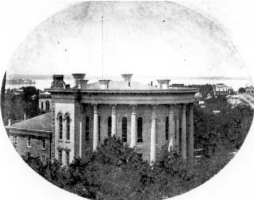
The first phase of the second Madison capitol is shown as it appeared around 1860. At the left is the original capitol, which would be torn down a few years later. (State Historical Society, #WHi (X3) 50748)
