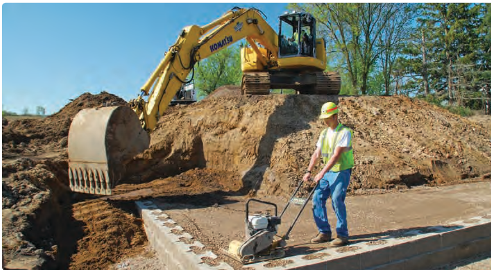
WIS 40, Chippewa County
