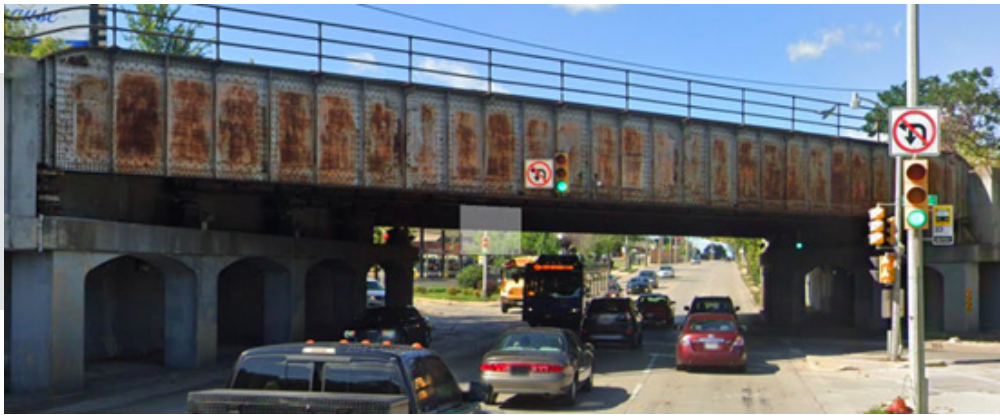
Figure 9. Fond du Lac Avenue and Locust Street, the intersection with the highest societal cost crash rate of any intersection in Milwaukee. Off-street pedestrian crossing proposed in this project will substantially increase safety and reduce the societal cost of accidents at the intersection.
