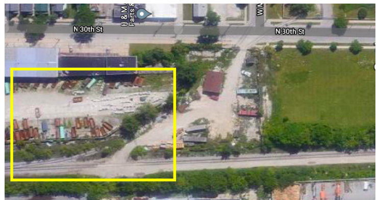
The parcel above, located just north of North Avenue, was once a utilized rail spur that is no longer active. Former rail spurs provide opportunities for new tenants within the Corridor
