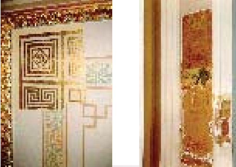
Paint probes uncover the decorative schemes for the capitol through the decades. (Gerilyn Schneider)
